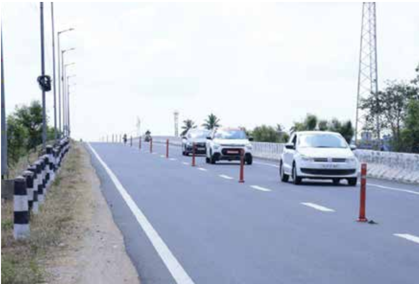
Figure 13.1: Bollards installed on the Kallakurichi Bypass Road to separate the opposing flow of traffic
