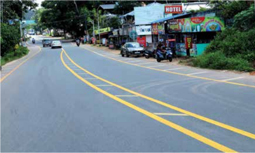
Figure 2.3: Hazard markings on the safe corridor (Source: KSTP-II/SCDP 2020)
