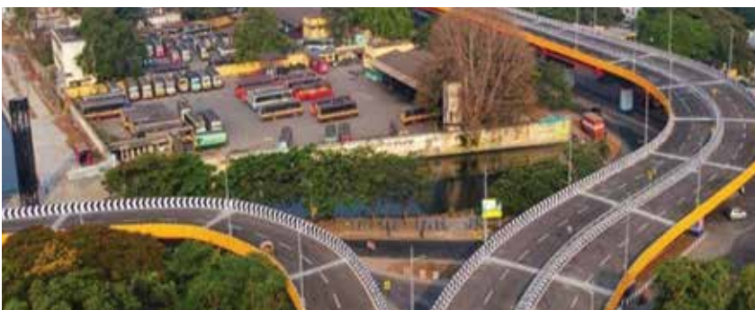
Figure 13.2: A flyover in Coimbatore lacking superelevation at curves
