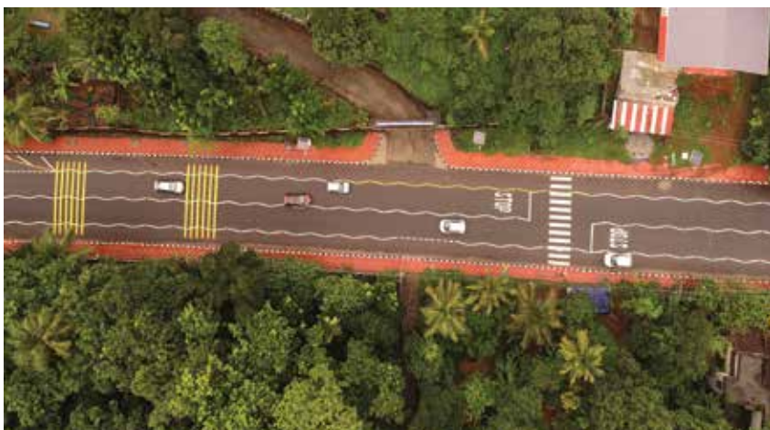
Figure 2.5: Aerial view of School Zone treatments carried out on the corridor (Source: "KSTP-II/SCDP" 2020)
