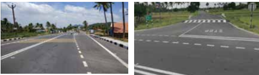
Figure 9.2: Installation of edge lines and raised pavement markings (Source: Srinivasan 2020)
