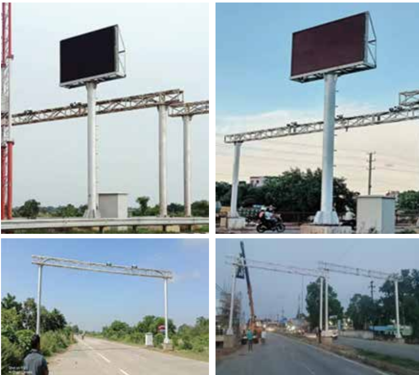
Figure 12.2 Electronic enforcement measures installed under the DEESHA project (Source: STA "DEESHA" 2023)
